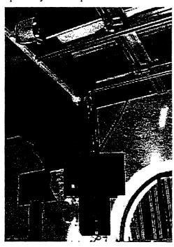
Each speaker hangs from a rotating beam. The pivot point for each speaker runs in a track that slides along rails bolted to the ceiling. With height adjustment of each suspension cable, this system safely allows speakers to be moved anywhere in the room and oriented along two of the three possible axes. Rotational symmetry of the concentric drivers in Meyer HM-1 speakers obviates the need for adjustments around the third or "roll" axis.
