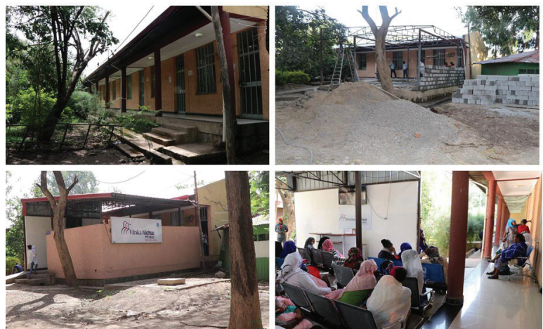
Renovation and Use of Adama's Michu Clinic
